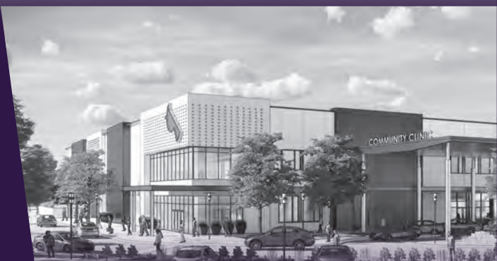
REDBIRD REDEVELOPMENT PROJECT | DALLAS, TX Floating Rate Renovation Loan 295,000 s.f. Mixed Use - Office & Medical
